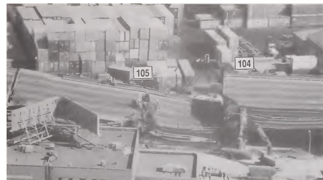
Damages of I-880 Cypress Structure in Oakland after 1989 Loma Prieta Earthquake
